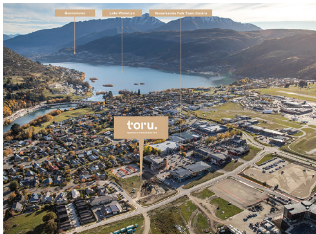
Toru Apartments in the heart of Remarkable Town Centre
