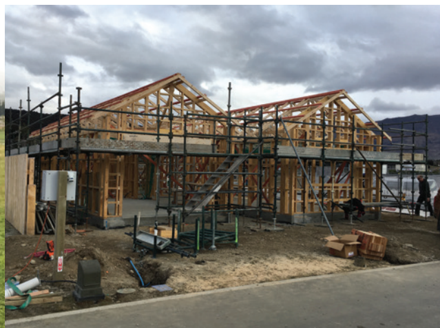
Homes under construction at Hikuwai, Wanaka
